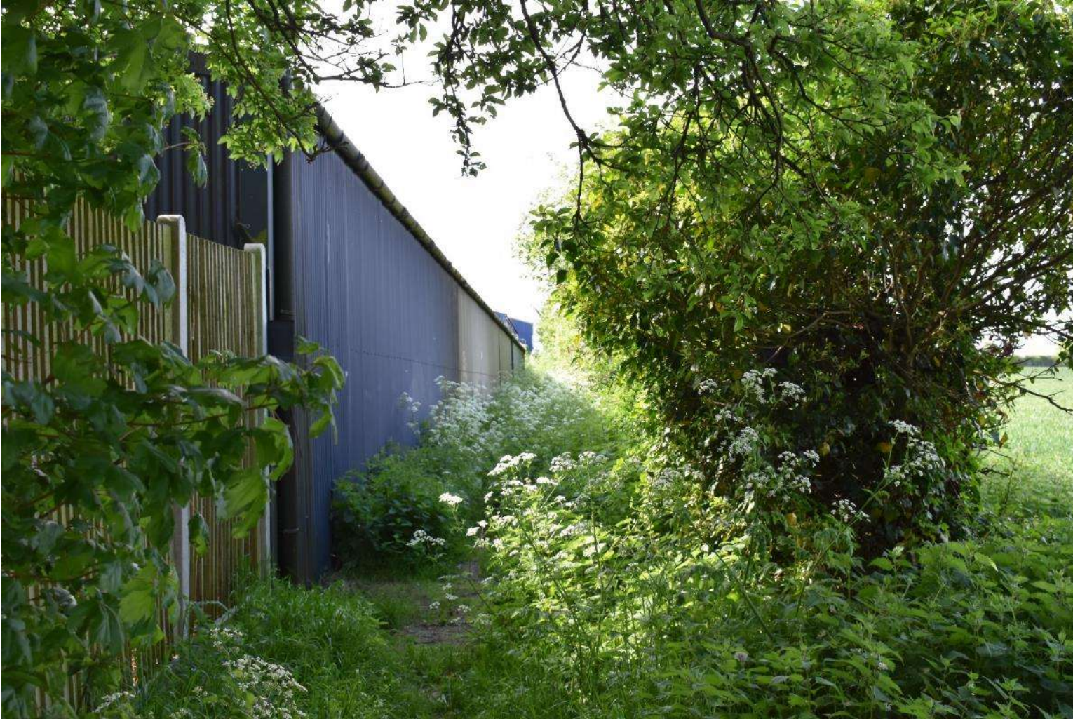
Plate 10: View along footpath at the northern boundary from current entranceway looking towards new entranceway area (facing NW).
